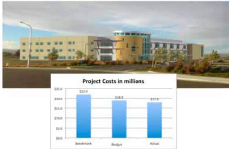
Figure 4. Sutter Fairfield medical office building (The Boldt Company 2008)
